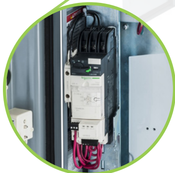
Starter in "Installation" position for easy access
